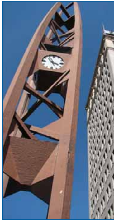
CLOCK TOWER & 1060 FULTON
